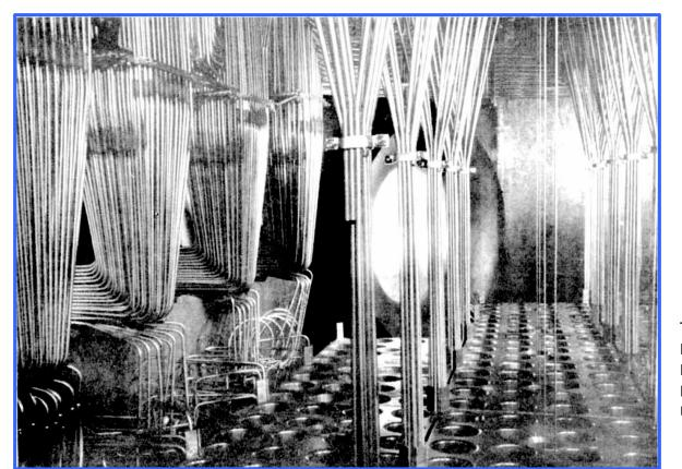
This and previous slide, Reactor Core Design Principles, Air-Cooled and Magnox, B. J. Marsden, The University Of Manchester.
